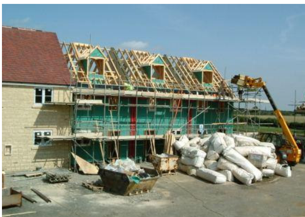
Eight new Eco-friendly homes under construction in Fritwell - September 2006
